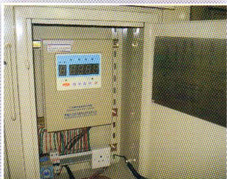
Winding Temperature Scanner
